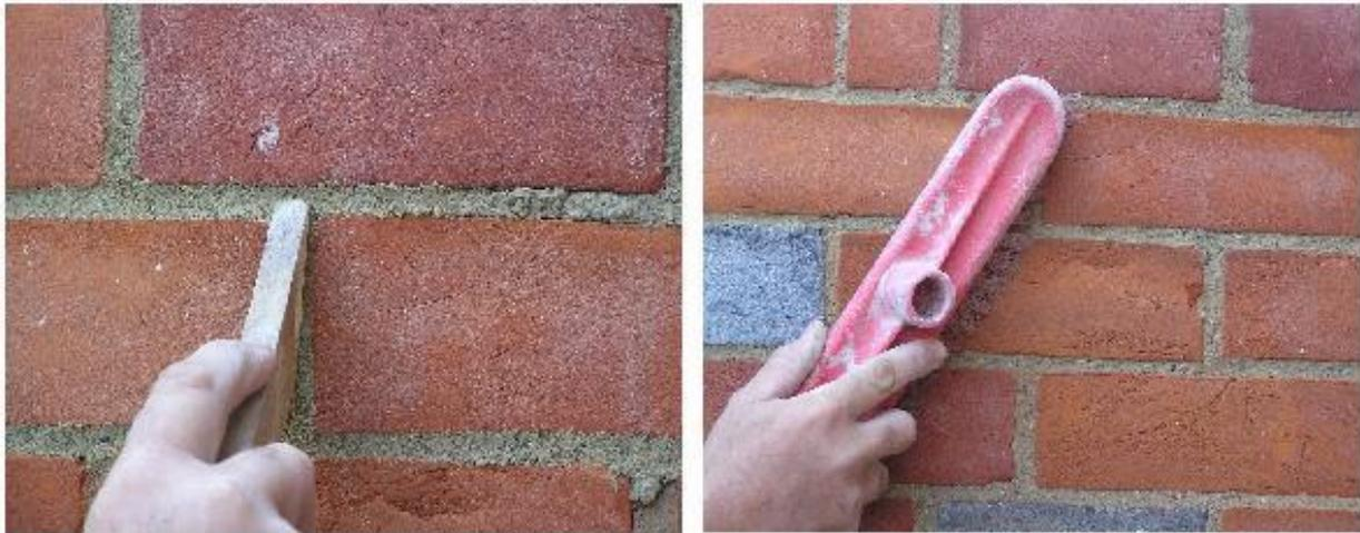
**NOTE:** If mortar gets onto the face of the brickwork/ stonework brush or beat it off when it is dry. Removal whilst the mortar is wet will spread staining. Stains can be removed using a mild brick acid however; the natural weathering process will remove most stains over the winter period.
